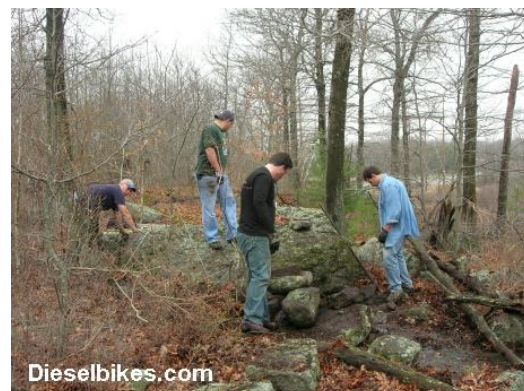
The Stone Bridge Crew—This was the toughest job.
